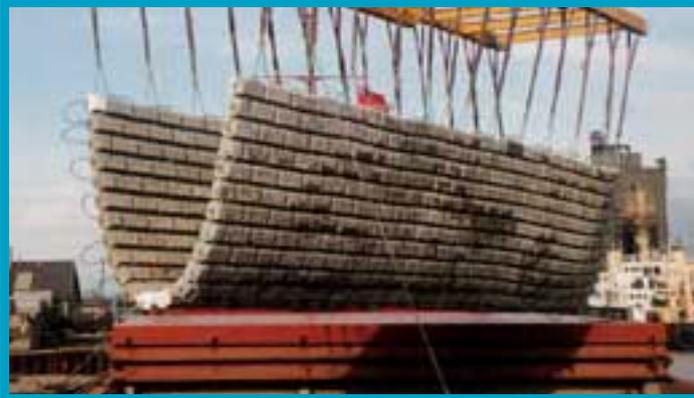
Plate 2.17 Concrete Mattress (Source: Submat/SLP Engineering)
