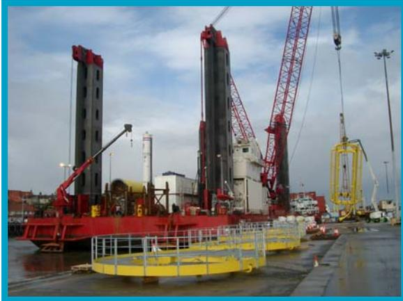
Plate 2.10 Loading components onto jack-up barge from quayside
